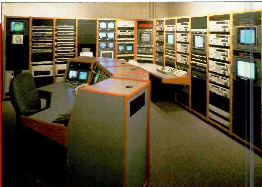
Network master control room. L-R rack No. 1--- fiber receive/transmit. Rack No. 2 and 3--- audio/video patching. Rack No. 4 --- character generation and control. Rack No. 5 --- network monitoring. Rack No. 6 (corner)--- engineering station and monitoring. Rack No. 7--- network record and playback. Racks No. 8-12--- commercial insertion.
