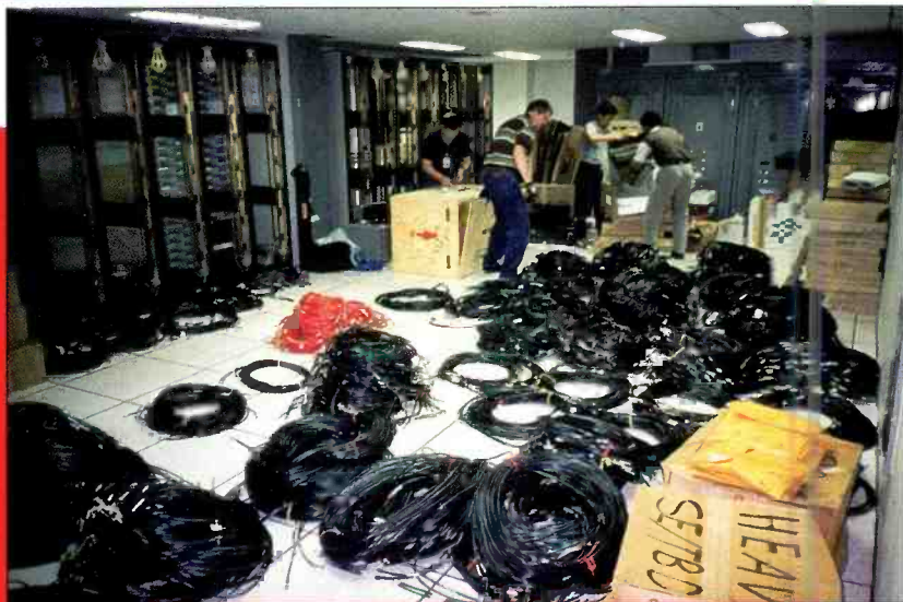
Cable installation in TV technical area. (Photo courtesy of Swiderski Electronics.)
