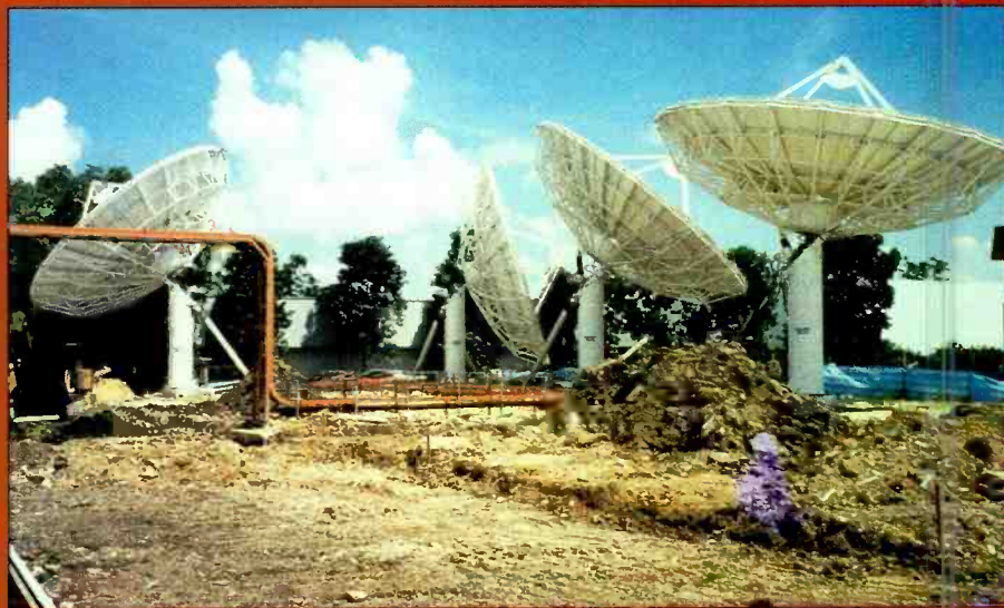
Satellite antenna farm. Note the disks have yet to be aimed.
