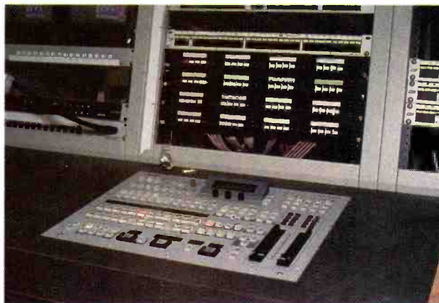
The central component of the new facility is the Sony serial digital master control switcher.
