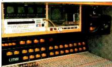
The Nashville Network's Remote Unit No. 2 uses a Telex/RTS ADAM system, an example of a digital matrix intercom using 4-wire analog audio paths to its stations.
